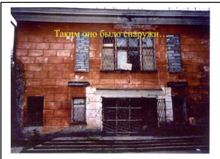
Exterior - Front (Before)
